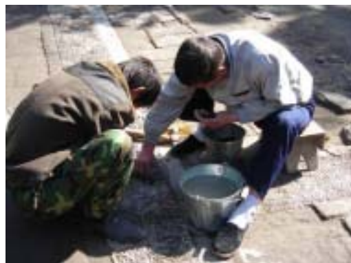
图 117 古建修缮工人正在维修“石子画”。 Fig.117 The worker who repair ancient building is maintaining “the gravel ground pattern”.
